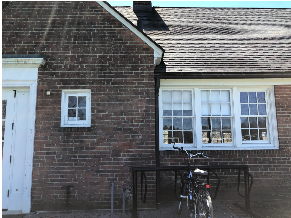
Figure 4.3: One of the Two Half-Size Windows (left) at the Field House
