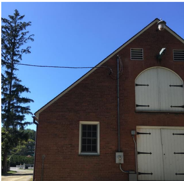
Figure 2. Side Shot of the Roof of Field House
