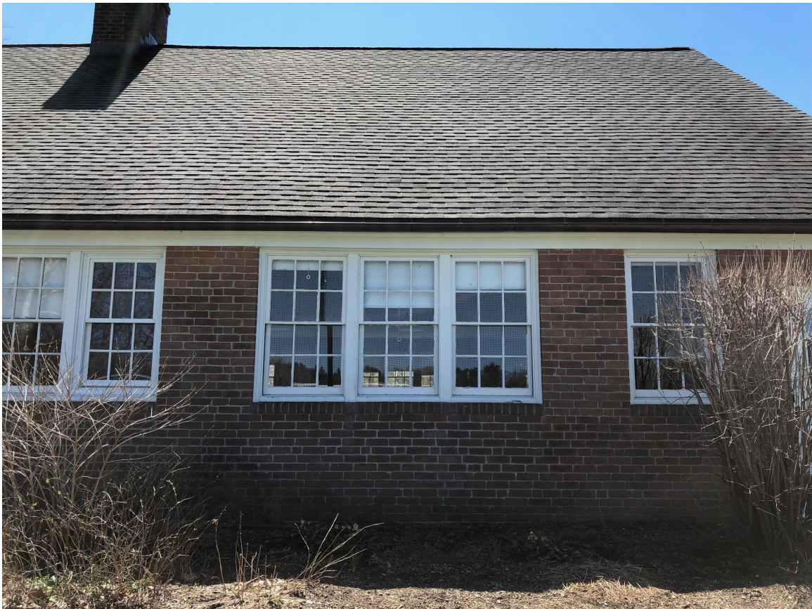
Figure 2.2: The Building Exterior of the Field House.
