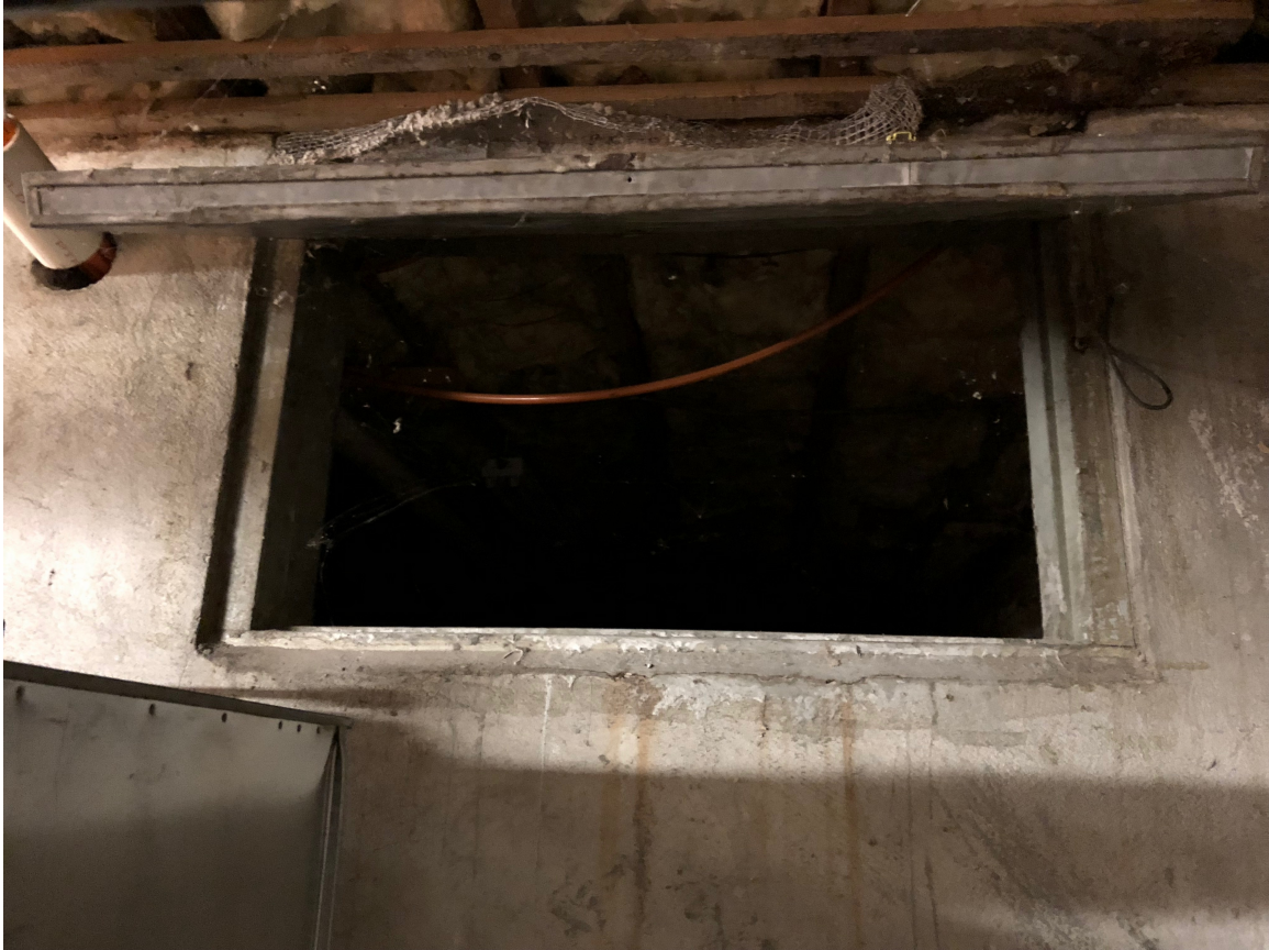
Figure 2.8: One of the Two Irregular Spaces in the Basement
